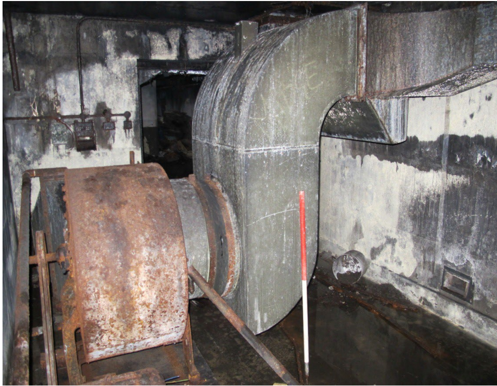
Figure 24: Shot of the air ventilation room G12, showing the central air handling unit for the building. Looking west.
