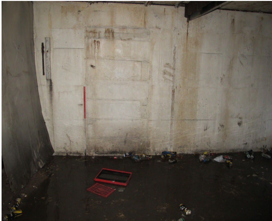
Figure 43: Detail of one of two blocked doorways located along the west wall of room F7. The doorway would have originally provided access to a walkway or room that ran around the top of the main operations room G4. Looking west.
