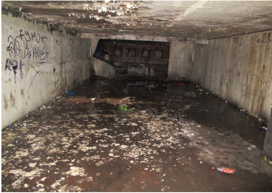
Figure 41: General shot of the short range shooting gallery in room F7, showing the metal sheeting of the butts area at the southern end of the room.
