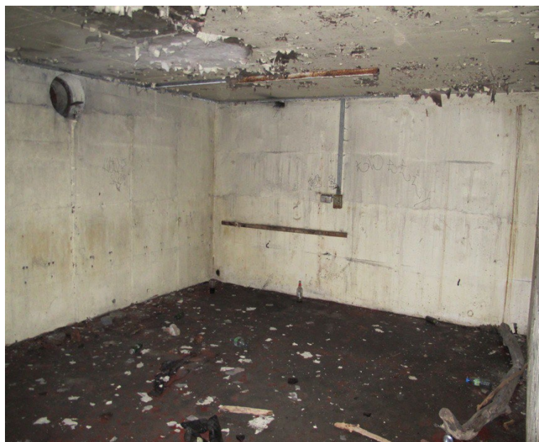
Figure 34: General shot of room F3 showing light switch on the north wall and an open air vent cut through the west wall. Looking north.
