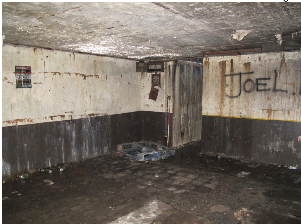
Figure 31: Detail of blocked southern stairwell S1 in room F1. The wooden hatch marks the location where the stairs would have risen to from corridor G1 on the ground floor.
