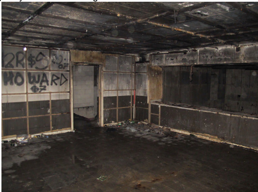
Figure 38: General shot of the viewing gallery room F5 showing the eastern doorway and the viewing window that looks down on to the main operation room G4. The walls and ceiling were found to be covered in wooden framing, a likely mounting for wooden panels. Looking southeast.
