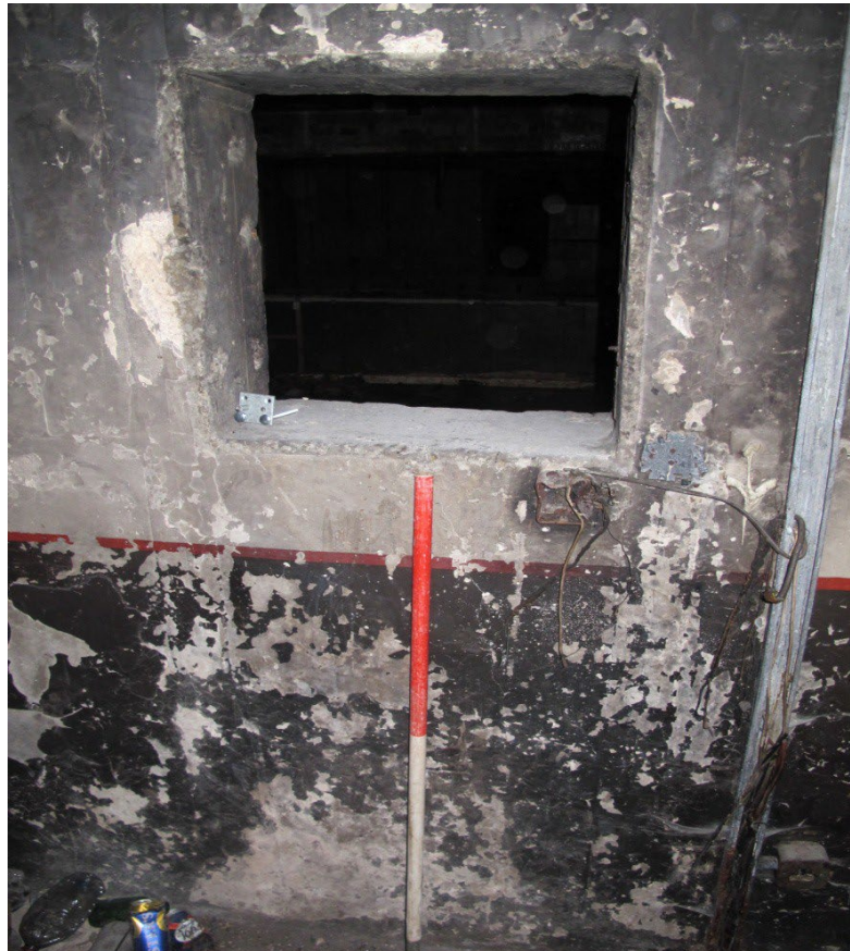
Figure 37: Detail of a window cut into the partition wall between corridor F4 and the viewing gallery room F5. Looking south.
