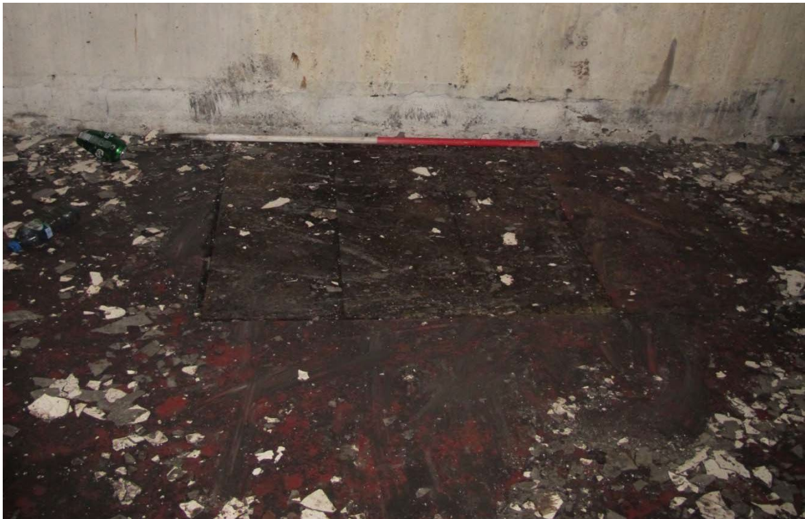
Figure 31: Detail of blocked southern stairwell S1 in room F1. The wooden hatch marks the location where the stairs would have risen to from corridor G1 on the ground floor.
