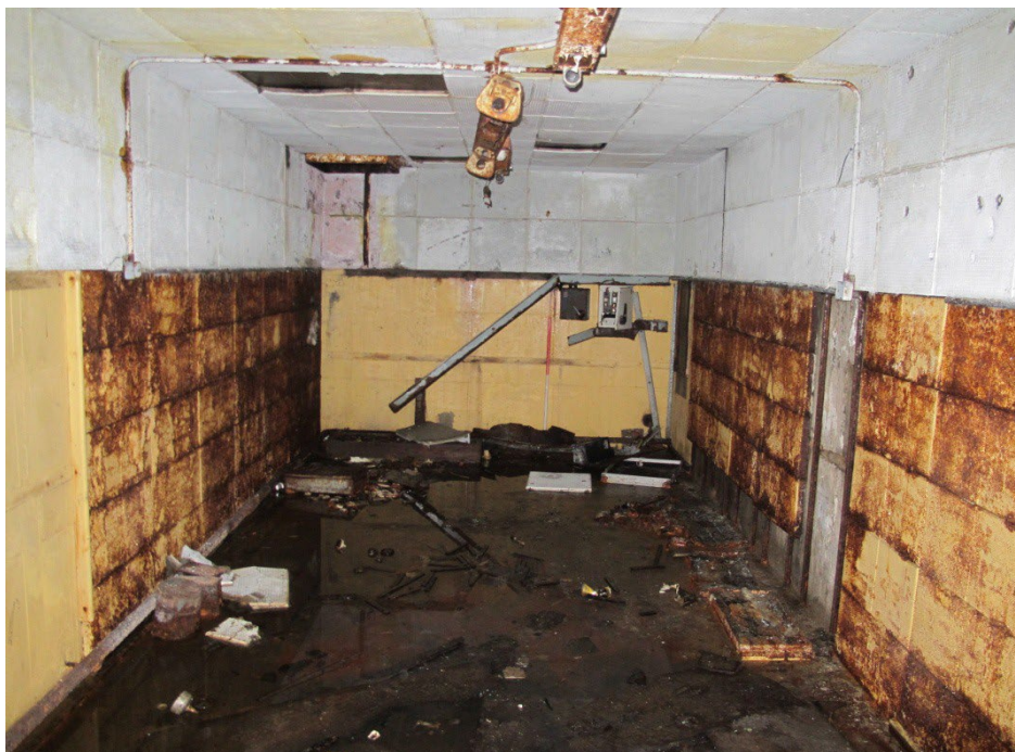
Figure 10: General shot of southwest radio control room G2 with sound proofing tiles covering the walls and ceiling. Looking west.
