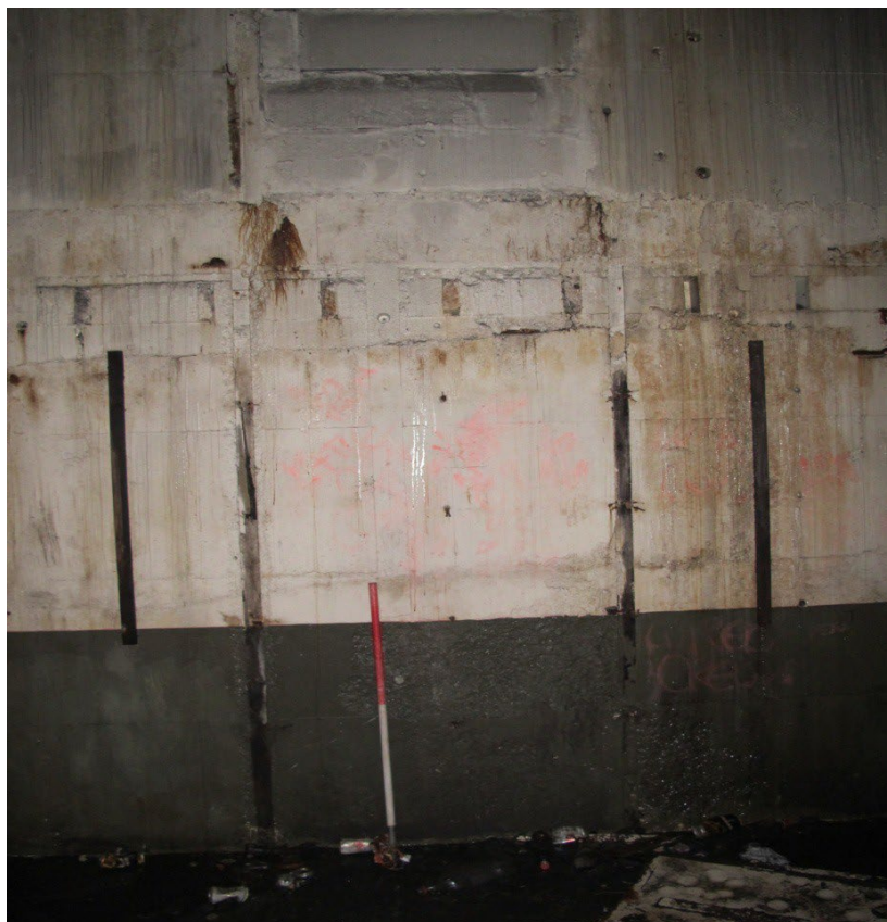
Figure 13: Detail of fixings for possible shelving on the east facing wall of the main operations room G4. Looking west.
