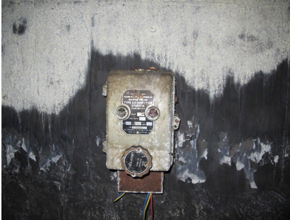
Figure 25: Detail of wall mounted control device for the ventilation unit in room G12. The device was fixed to the south facing wall of the room.
