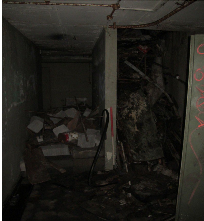
Figure 9: General shot of corridor G1 with blocked staircase S2 to the right. Looking north.
