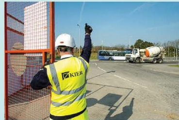
CLOCS trained gate marshal
